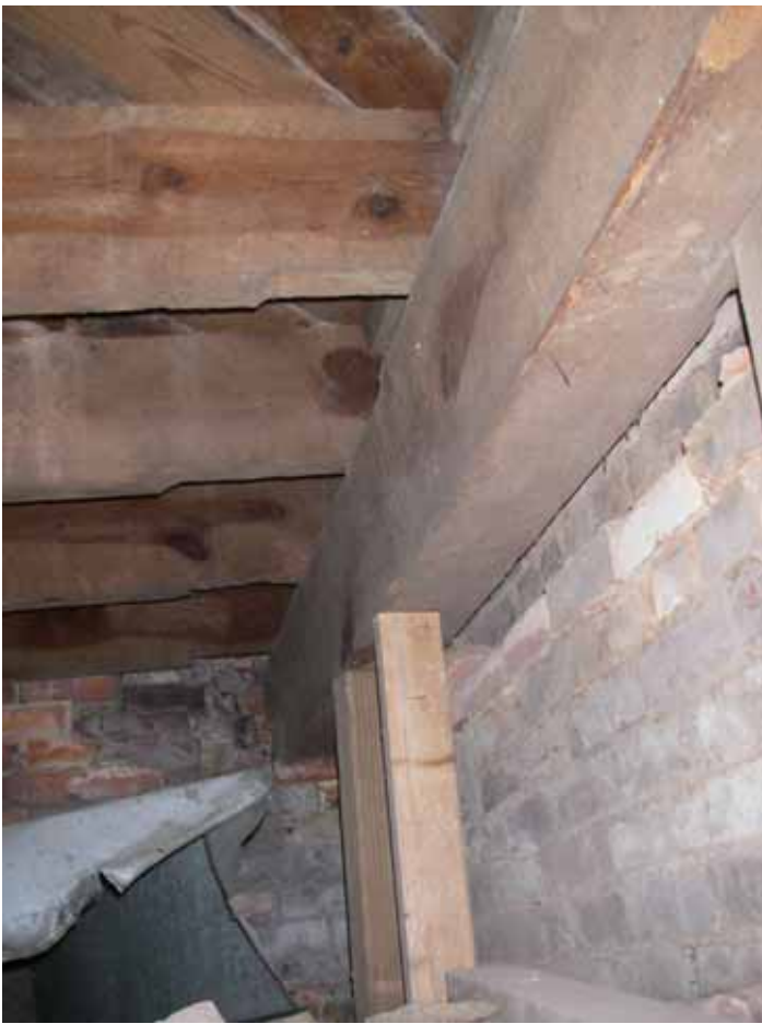
Photo #38 This picture shows the right/rear corner of the transept, where more temporary shoring was added. In many ways, this area is a mirror of the left/rear transept seen in photos #30 through #33, with the exception of wood having been used to support the 6x10 girder. See the following for additional description.
