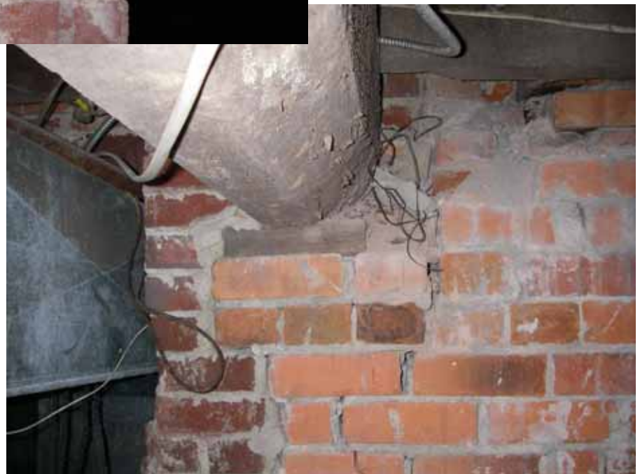
Photo #26 This picture shows the back end of the 6x10 (with considerable wane at its right bottom edge). The brick supporting the girder is distressed. Large separations are visible at both the bed and head joints.
