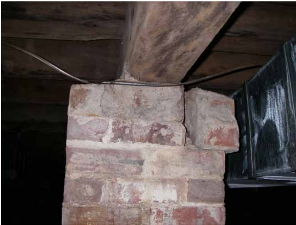
Photo #26 This picture shows the back end of the 6x10 (with considerable wane at its right bottom edge). The brick supporting the girder is distressed. Large separations are visible at both the bed and head joints.
